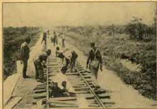
Workmen Laying Plank Between Rails Preparatory to Mr. Murphy's Famous Ride.
